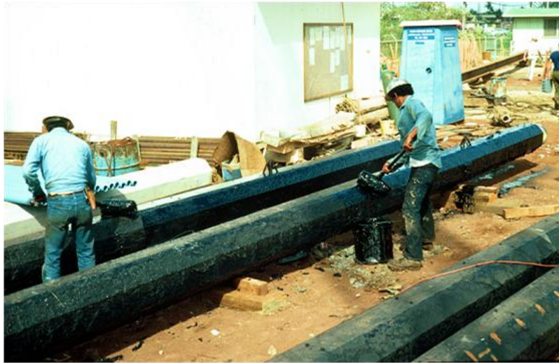
Fig. 7.49 View of applying a bitumen coat to a concrete pile
