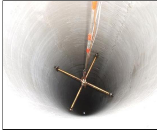
Fig. 8.23 A Glostrex anchor placed down in a cylinder pile (Hanifah and Lee 2006),
