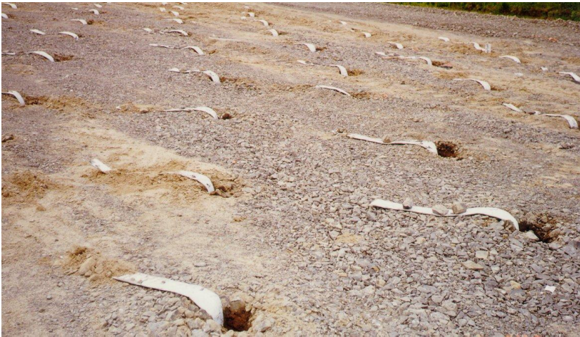
Fig. 4.9 View over a site after completed wick drain installation
