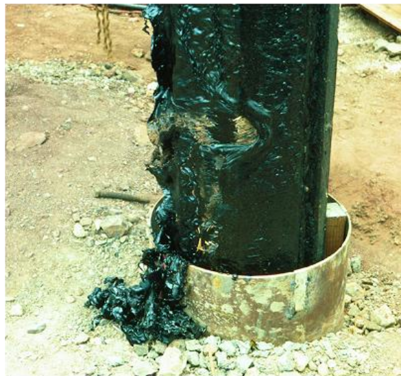
Fig. 7.50 View of a bitumen-coated pile driven through a protective casing The left side of the pile was the pile underside in storage
